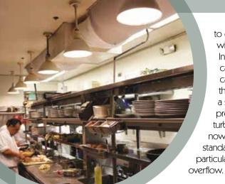
to distribute air throughout the 1,000-square-foot kitchen, the diffusers were replaced with two eight-foot-long, 28-inch-diameter D-shaped KitchenSox® fabric diffusers. Instead of the metal diffuser's estimated 500-fpm airflow that
