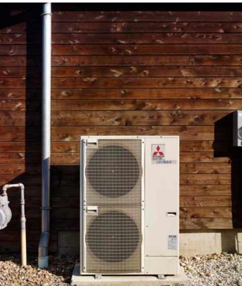
The Mitsubishi Electric VRF zoning system is able to provide the home with the flexibility to cool and heat only those rooms that are needed. An access panel to an indoor unit provides easy serviceability and is located discreetly on the back porch of the home (pictured right).
