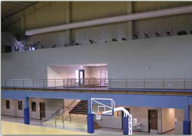
Maintaining air comfort on the second floor perimeter running track was an air distribution challenge as well. While the 200-foot-long ducts condition the track on each long side, the building's shorter end caps are independently supplied each with a 100-foot-long run. One end supplies the third floor mezzanine cardiovascular workout area and has factory-engineered orifices that allow the air to evenly spill down to the track on the second floor.
