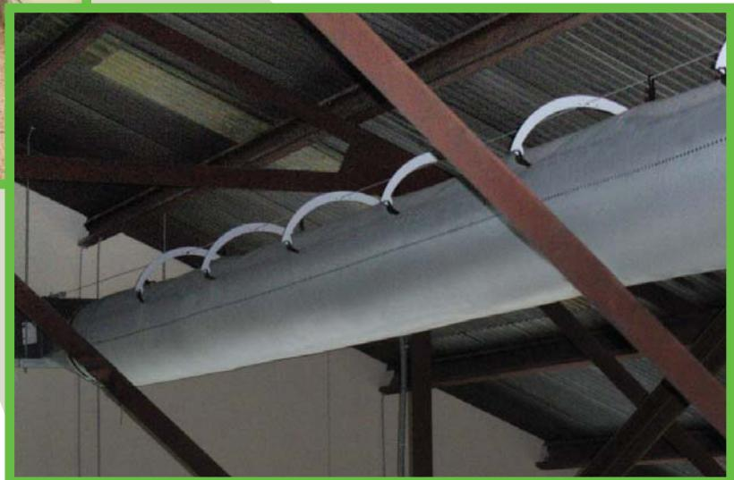
uses Comfort-Flow technology which allows approximately 15 percent of the air to actually flow through the fabric's factory-engineered permeability. Comfort-Flow also eliminates dust from accumulating on top of the duct thus providing better IAQ, according to Scott Spiva, sales engineer for manufacturer's representative, Texas Air Products, San Antonio, who helped specify the product.
